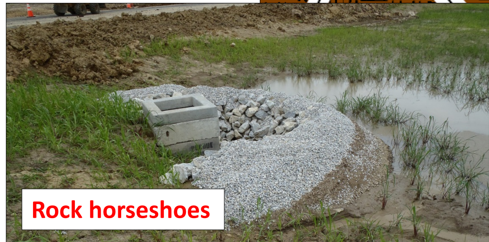
Perforated risers with filter pack
