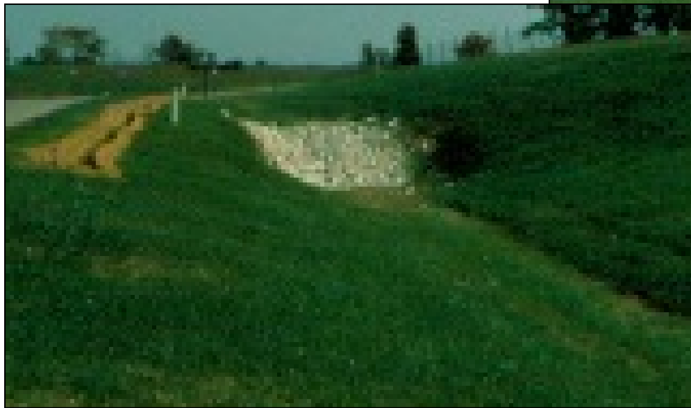
After (rock chute stabilized grade transition)
