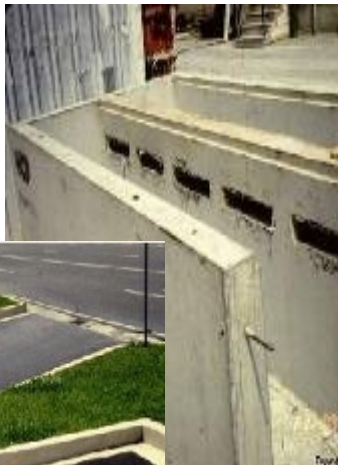
Perimeter Sand Filter
