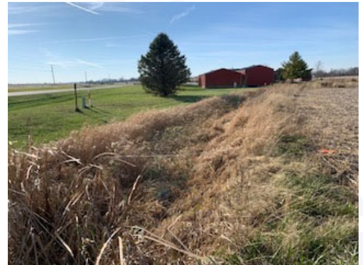
Dry Grass Swale, Hendricks County, Indiana
